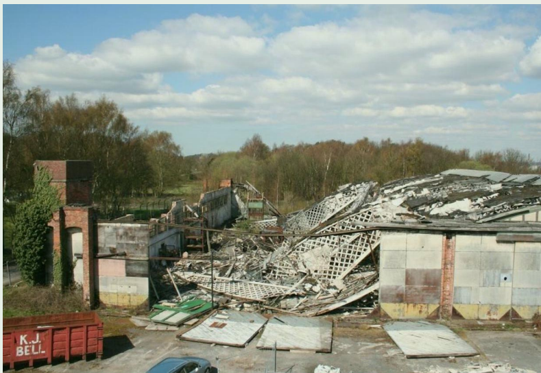
Hangar 16 before renovation.
